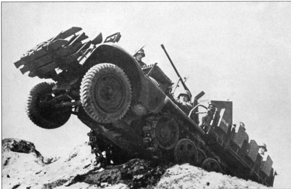
This impressive shot shows an unarmored Sd.Kfz. 10/4 combat vehicle negotiating a slope. The 1-ton halftrack was a most versatile vehicle. The version here, which is armed with the 2cm Flak 38 gun, quickly became famous as the Sturmflak - the anti-aircraft assault vehicle.
