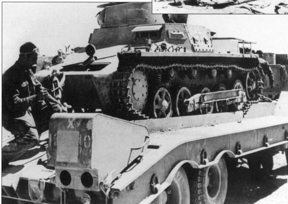
This Pz.Kpfw. I is being loaded onto a flatbed trailer for transportation to a vehicle dump. With the production and arrival in North Africa of heavier and more powerful models of German AFVs, the Pz.Kpfw. I became more and more outclassed. The vehicle looks undamaged and will probably be sent home for evaluation.
