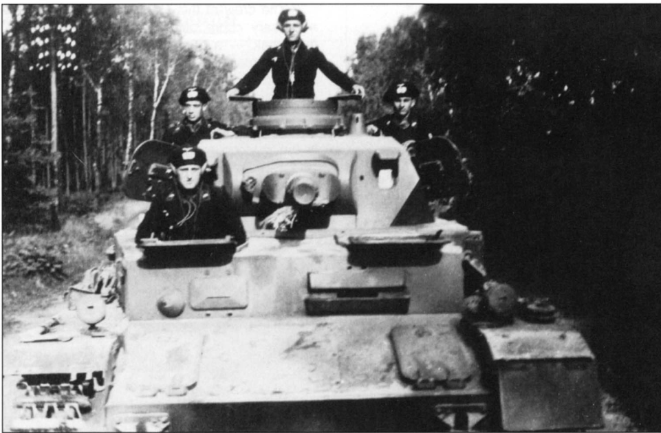
Used in the fourth and eighth companies, the Pz.Kpfw. IV tanks served as attack support vehicles. Armed with a 7.5cm L/24 gun, they would survey the battlefield and fight against enemy gun positions and heavy tanks. Except for the driver, the entire crew of this Ausf. B is visible at their hatches.
