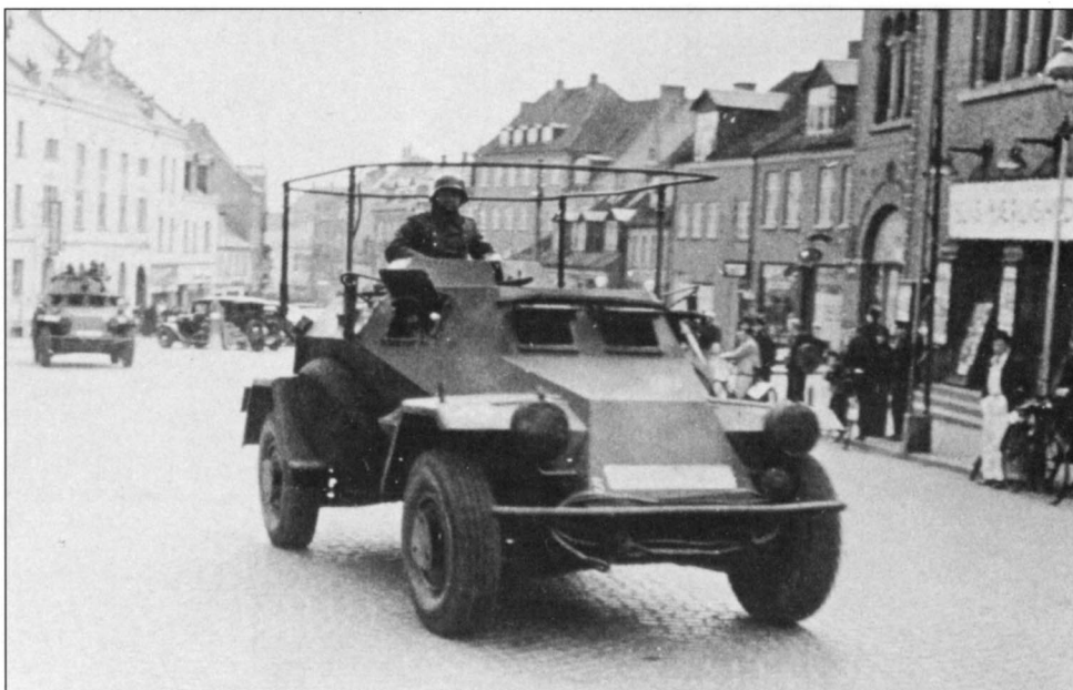
A Sd.Kfz. 223, followed by a Sd.Kfz. 222, passes through a French city. These armored cars were fitted with a large frame antenna, as most command and liaison vehicles were until 1942. Though effective, the conspicuous antenna attracted enemy attention, resulting in relatively high losses. Note the small number "5" next to the registration plate.
