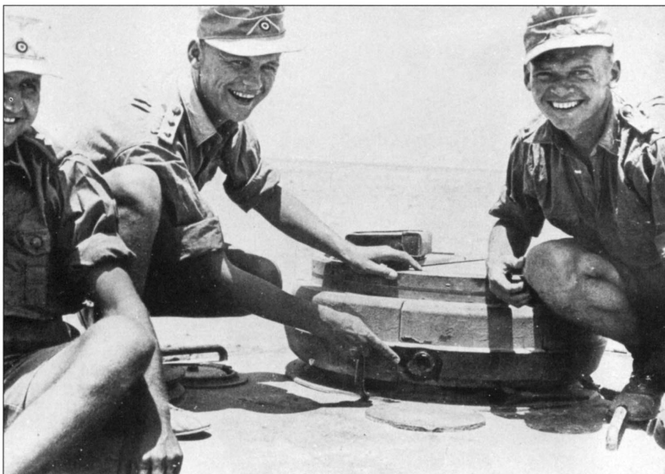
Smiling at their good fortune, Afrika Korps panzer troops take some time after a battle to pose for a photograph and point out where a British 2-pounder shell, which is still stuck in the cupola, had struck their tank. This photo was taken near Tobruk in September 1941.
