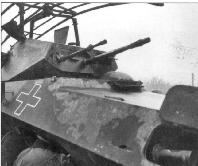
This Sd.Kfz. 232 Sechsrad (six-wheeler) was destroyed by a number of antitank rifle rounds. These old vehicles were phased out after the Polish campaign with only a few surviving in staff sections. Their cross-country performance and armor protection were never sufficient. Of interest is the German cross, whose inner portion has been neatly painted gray to discourage enemy gunners from using it to target the tank.
