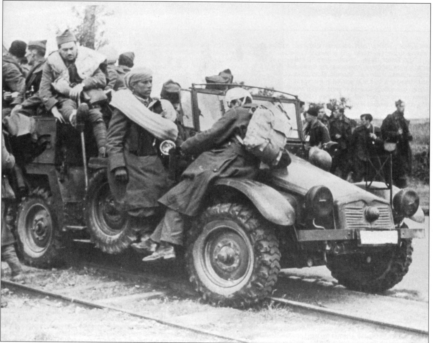
This overloaded Krupp-Protze light wheeled vehicle is transporting POWs, among them some colonial soldiers, to a camp. Although very useful and reliable, these vehicles suffered from limited cross-country abilities since they lacked a driven front axle.
