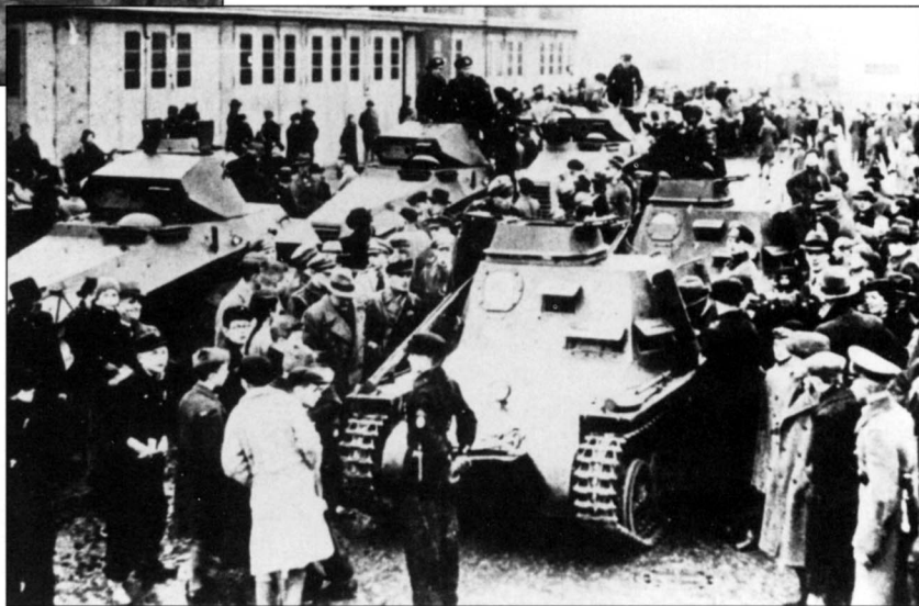
Photographed shortly before the Polish campaign, these early Pz.Kpfw. I Ausf. B kleine Panzerbefehlswagen (small armored command vehicles) still lack their machine guns. The aperture for the gun, which is located just below the small cupola, is sealed by a steel plate. Command vehicles were available in large numbers and played an important part during the advance of the German tank force during the Blitzkrieg.
